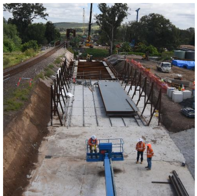
Photo: casting yard
