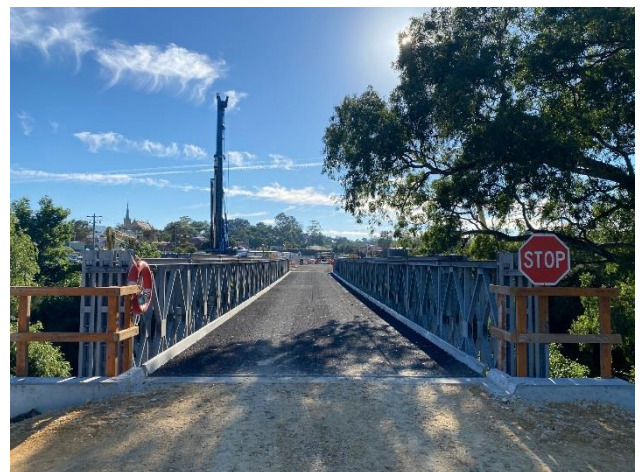
Photo: Temporary construction access bridge over Muscle Creek
