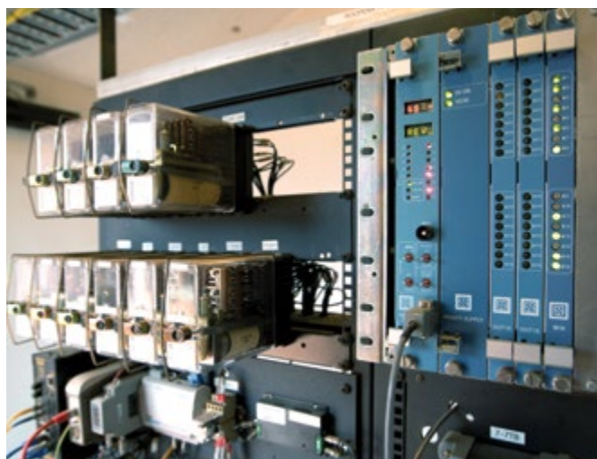
Figure 12: Track Interface Unit
