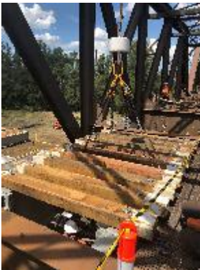
Image 3 - Replacement of bridge stringers during a previous shutdown.
