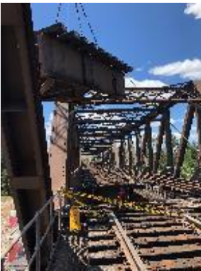
Image 2 - Removal of bridge stringers during a previous shutdown.
