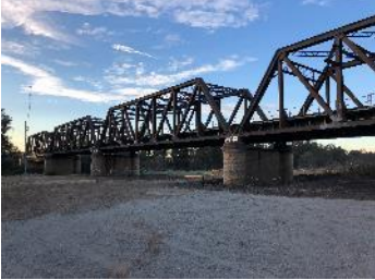
Image 1 - Stringer replacement works will be undertaken at Glennies Creek Bridge.
