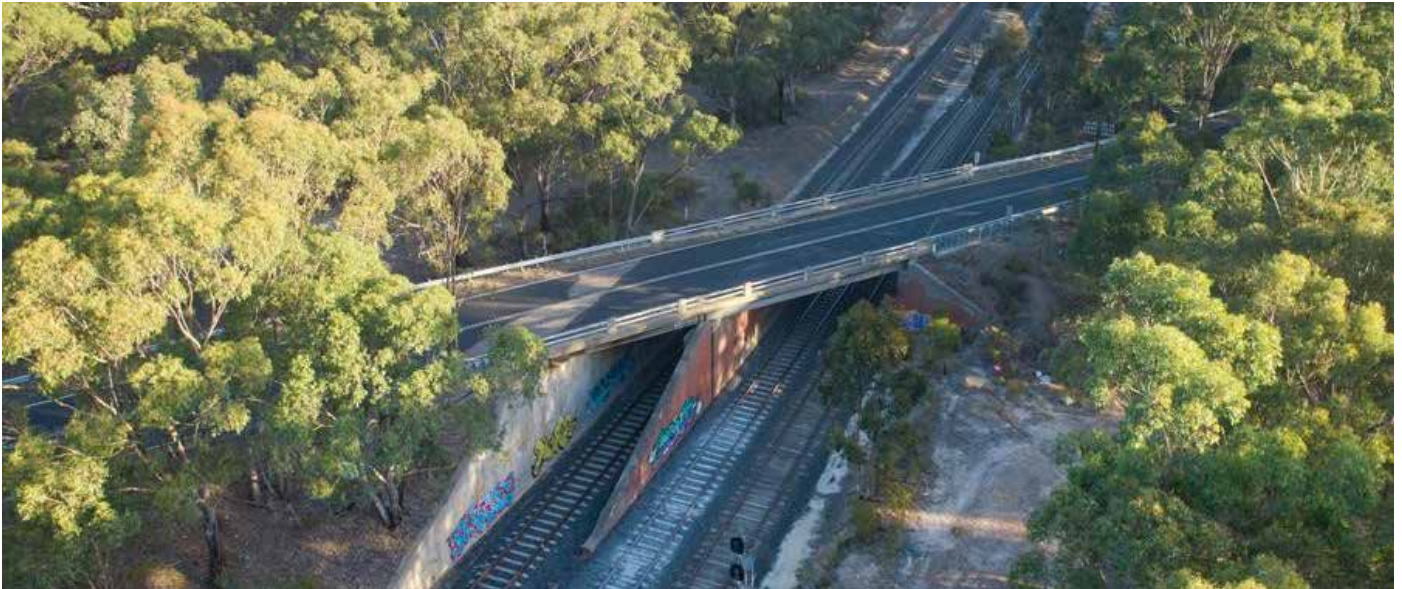
Seymour-Avenel Rd Bridge, Seymour is in the first tranche of works for T2A.
