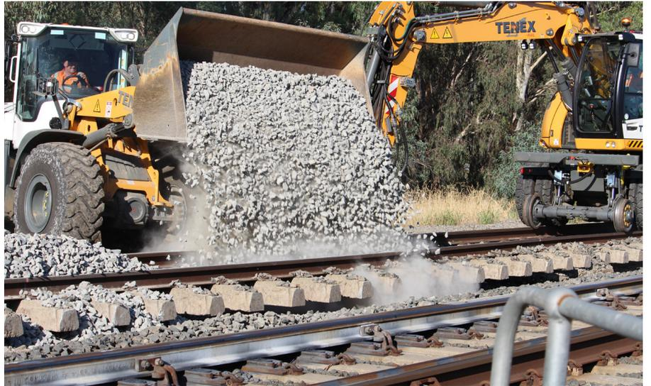
557,000 tonnes of locally sourced ballast has been used on the North East Rail Line Upgrade. New ballast has improved track stability and drainage, helping prevent new mud holes from forming.
