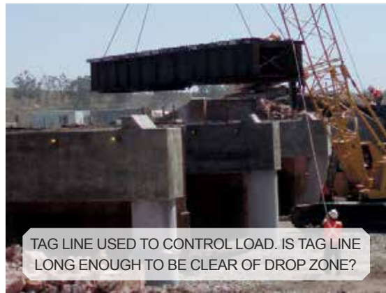
INSPECTED AND TAGGED LIFTING GEAR
