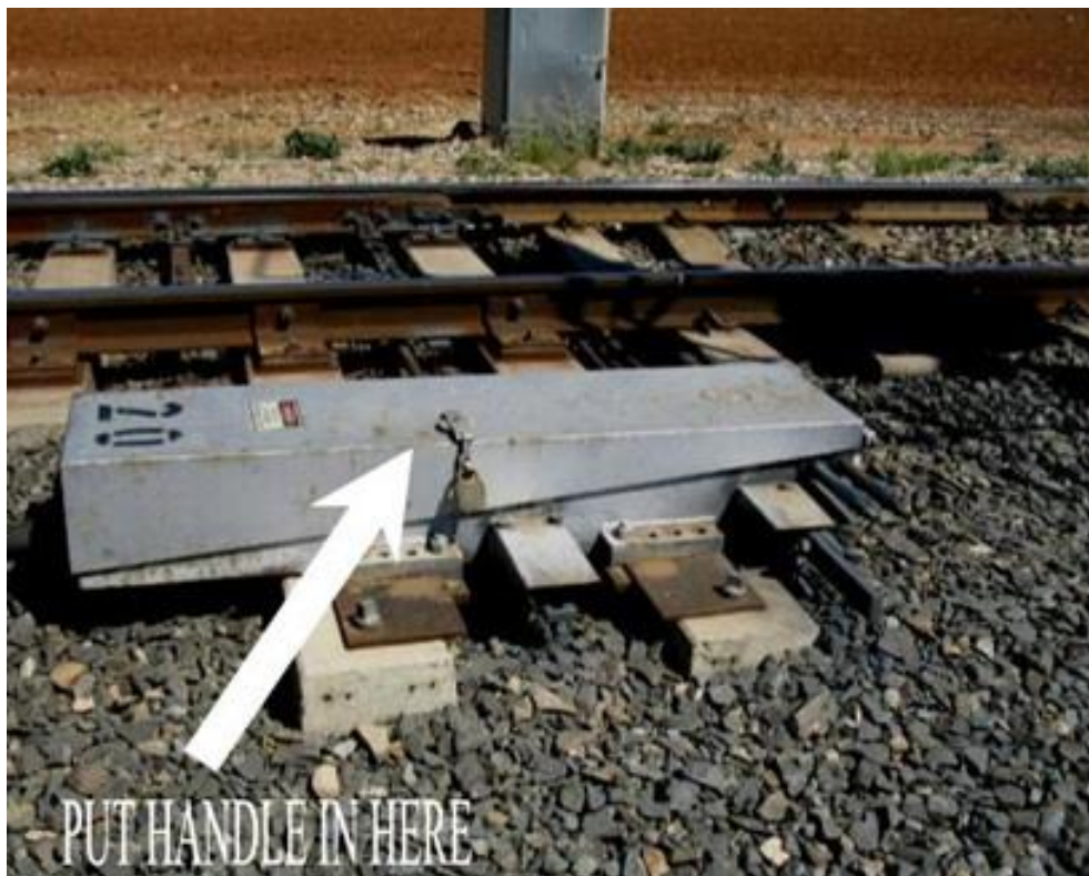
M70 points machine as used at no 5 points Mile End.
