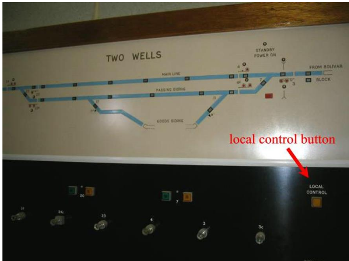
Two Wells local control panel in relay room.
