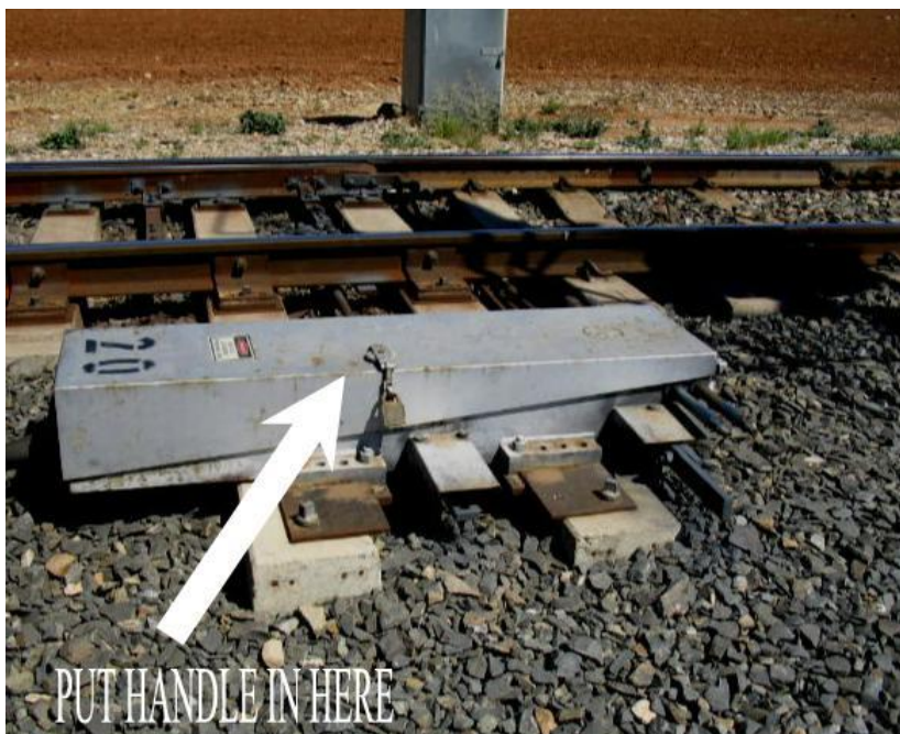
M70 points machine as used in West CTC.
