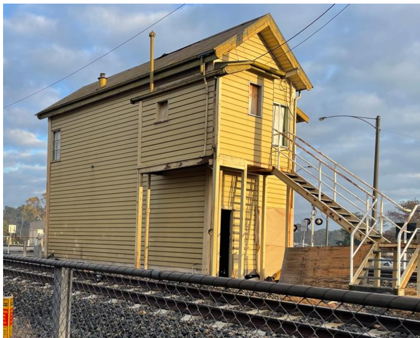
Figure 3-3 – Benalla Signal Hut (South-East corner)
