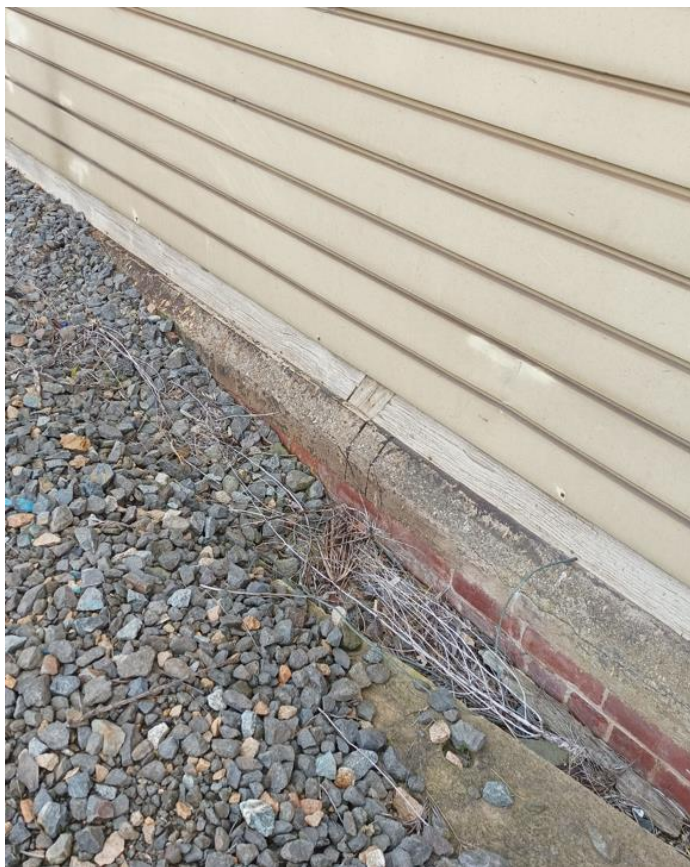
Figure 3-31: General photo of concrete footing on masonry bricks
