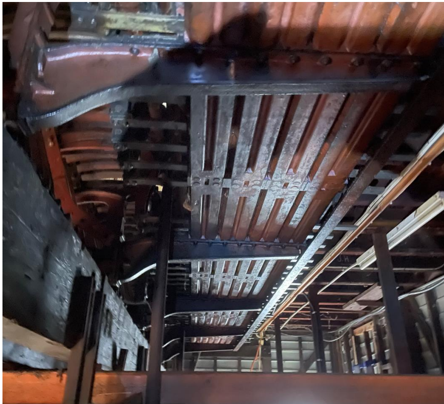
Figure 3-34: Signalling lever frame and associated equipment
