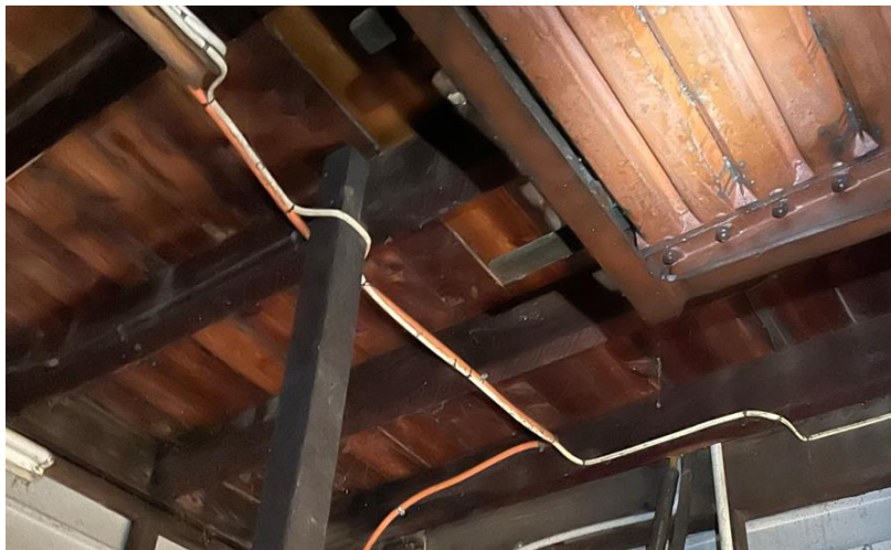
Figure 3-25: Underside of timber beams and deck flooring of the first floor
