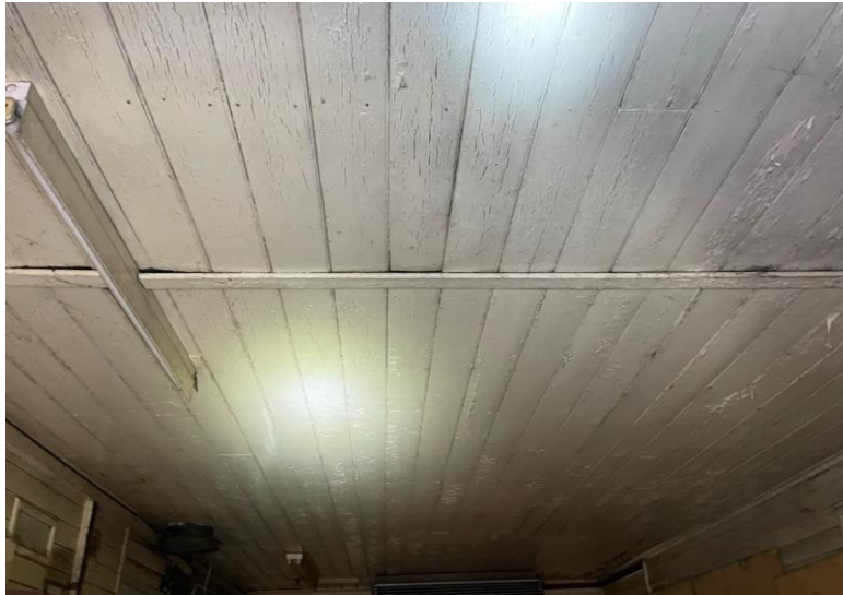
Figure 3-30: timber ceiling to first floor
