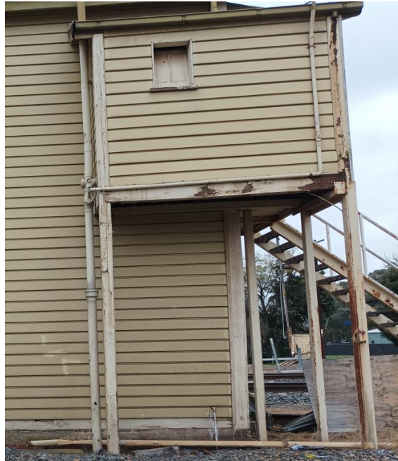
Figure 3-19: Non horizontal external beam supporting first floor toilet
