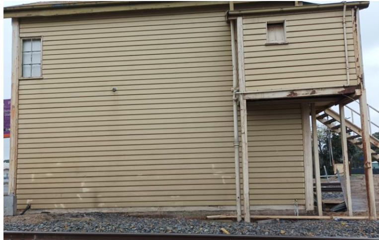
Figure 3-6: General condition of steel weatherboard cladding
