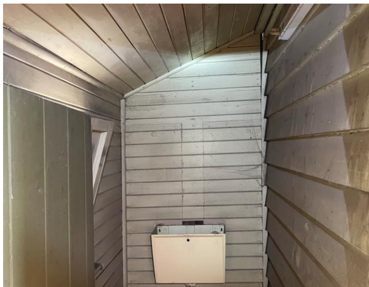
Figure 3-28: Timber walls for first floor toilet
