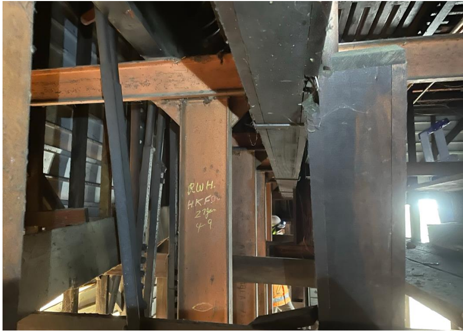
Figure 3-41: Internal steel lever frame supports
