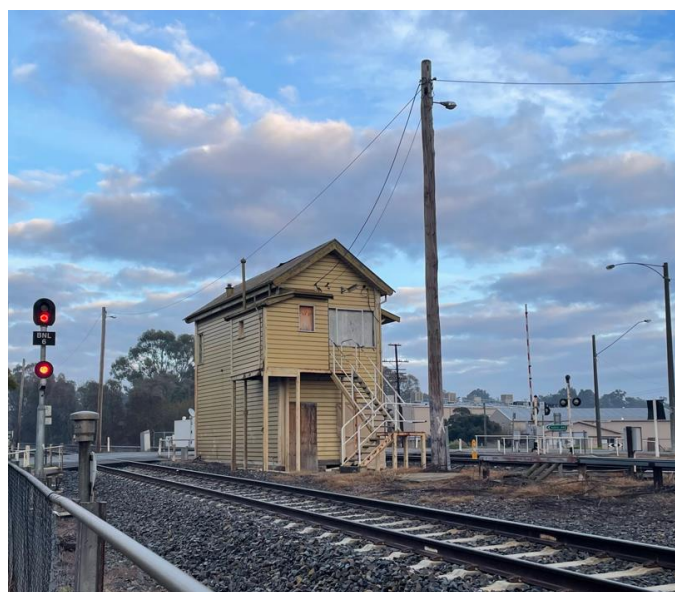
Figure 3-2: Benalla Signal Hut
