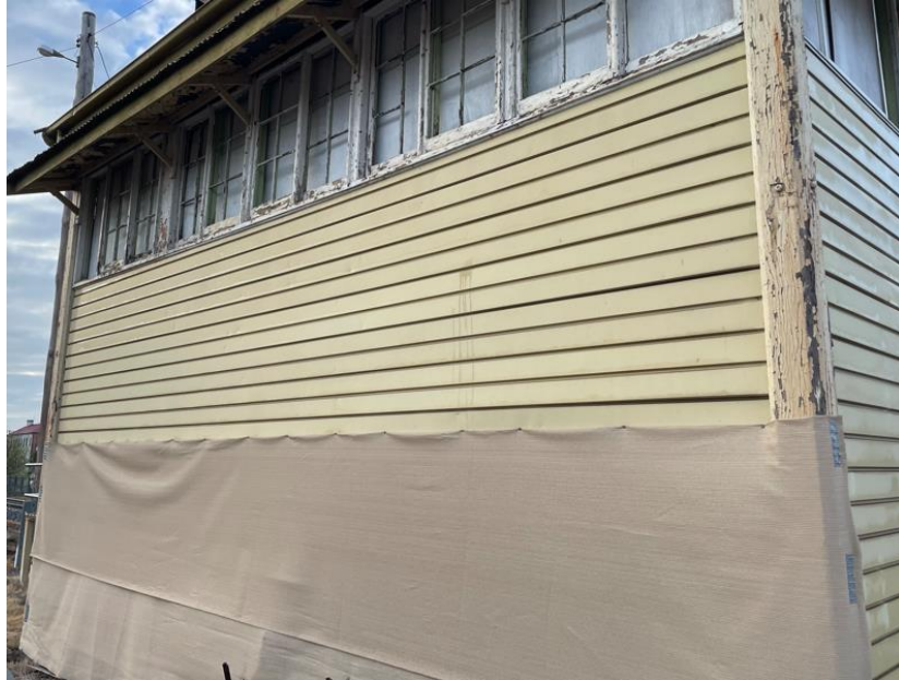
Figure 3-4A – Benalla Signal Hut (North West Corner)
