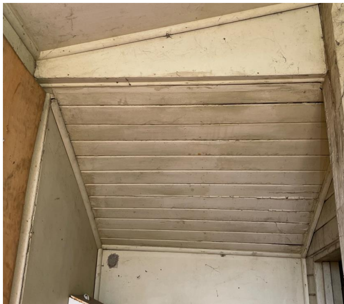
Figure 3-27: Timber ceiling adjacent to first floor toilet
