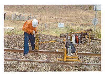
The Dog Spike puller, Fast clipper and E-clipping machines supplied to TEJV have no braking system and these are a standard piece of equipment used in the rail industry that are supported by trolleys.
