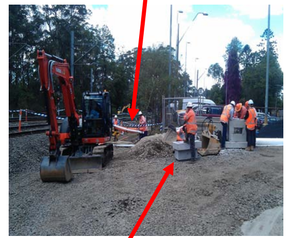
Location of Geotech Engineer before the incident
